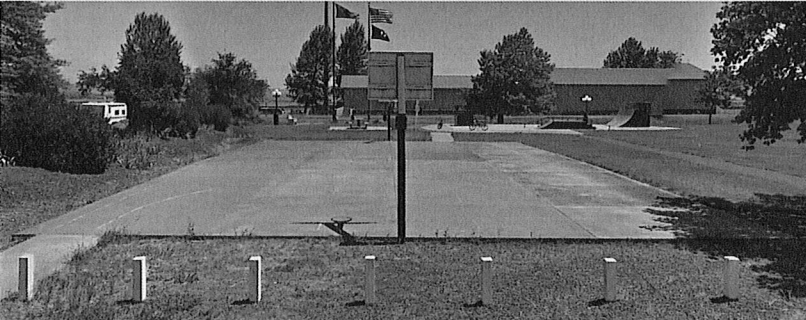
Concrete court with faded lines and non-adjustable hoops.
